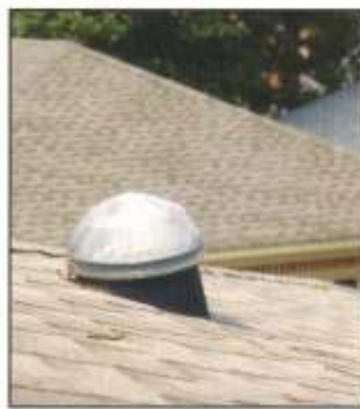
In addition to making use of as much natural light as possible, Cindy and Richard Wallace's EarthCraft home is designed with energy-saving features such as "The Energy Detective" (TED) energy monitor, top, and a light tube in one of the bathrooms, above.
